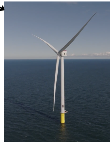
WIND TURBINE GENERATOR
